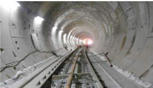
Mass Spring System Concreting in progress between Shenoy Nagar station & Pachaiyappa's Station
