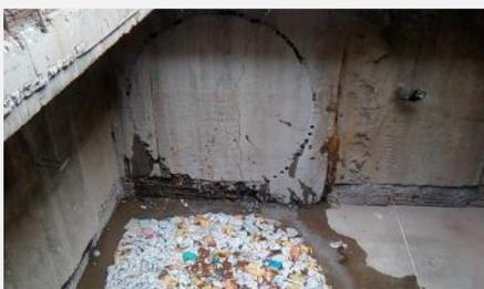
TBM 1 of UAA 03 package had a successful breakthrough at AG-DMS underground station. This TBM has completed tunneling of 2868mt from Saidapet to AG-DMS . One tunnel is fully completed between Saidapet and AG-DMS.
