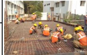
Rebar work in ground level slab of ancillary building at Nehru Park station
