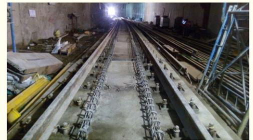
**Track concreting in progress between Saidapet ramp to Saidapet station**
