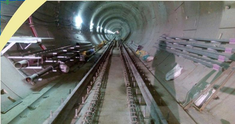
**Track concreting in progress between Saidapet ramp to Saidapet station**
