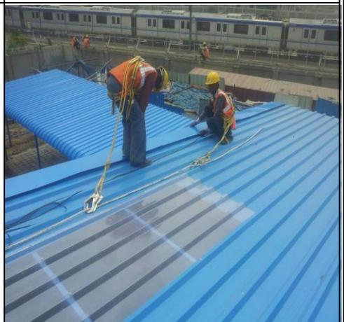
Uses of Life lines and mobile grab fall arrester for roof sheeting work.
