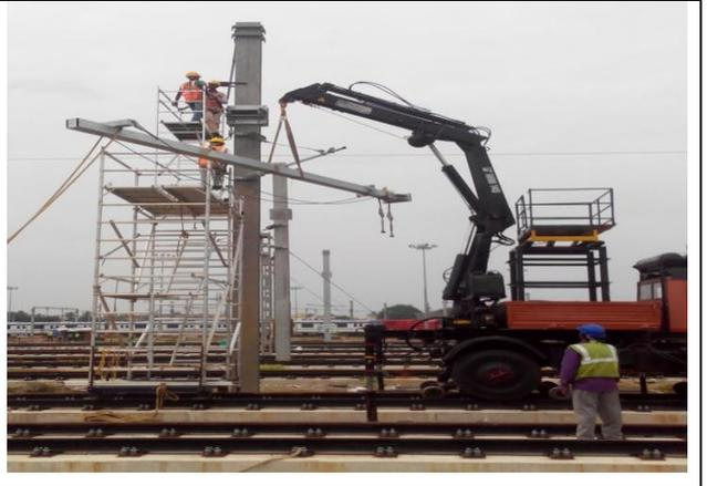
Two track cantilever erection using Unimog and trolley
