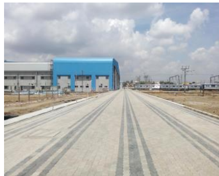
Paver works in front of stabling area
