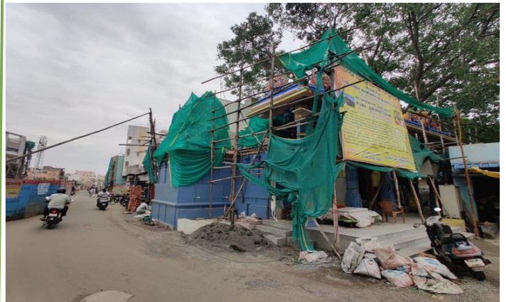
Kali Amman Temple, Kalyamman Koil Street — preserved through the realigned metro viaduct route
